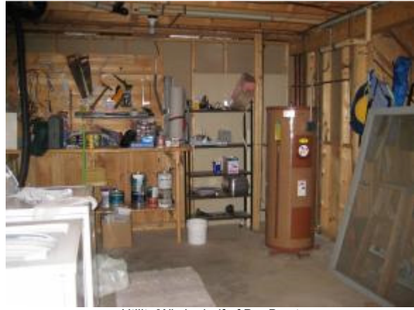
Utility/Wkshp half of Dry Bsmt
