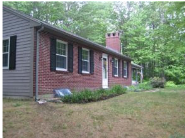
No Maintenance Brick Front
