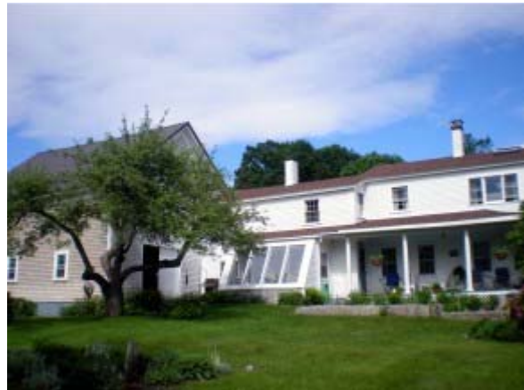
Two story barn, sunroom, porch
