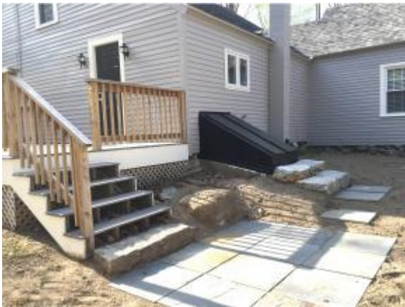
Back Patio & New Bulkhead
