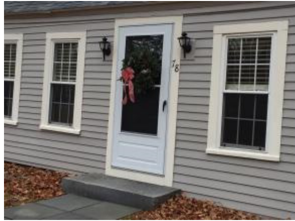
New Storm Doors
