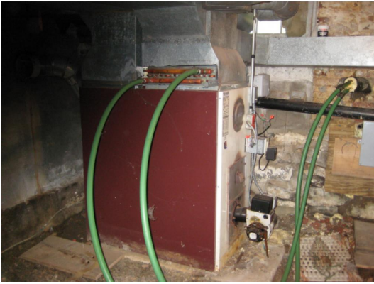
external boiler to FHA heat
