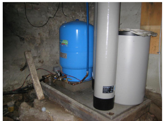
...and wellwater pressure tank
